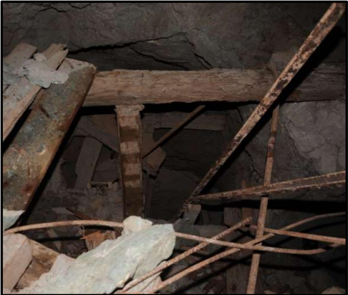
“Thursby” incline a double compartment winze on the tunnel level of the Higgins mine. The left compartment was a manway and pipe. A hoisting compartment was on the right.
