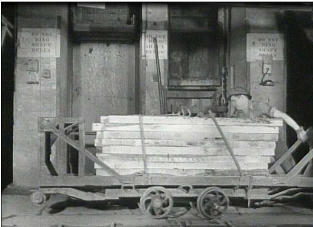
A Material Carrier after being unloaded from a cage at the Junction Mine C. 1930
